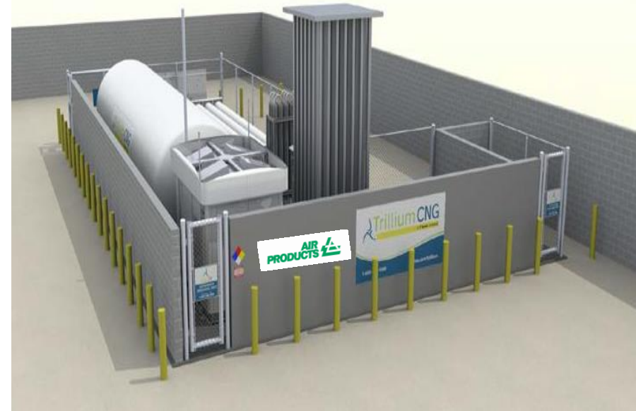
OCTA Hydrogen Station 30 kg per vehicle in 6+ minutes • From 2 dispensers simultaneously • Up to 1,500 kg/day
